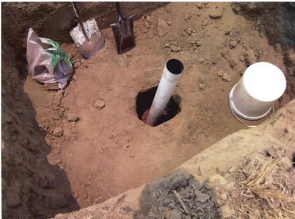
Figure VII.17. Photo of Percolation Test Pit.
