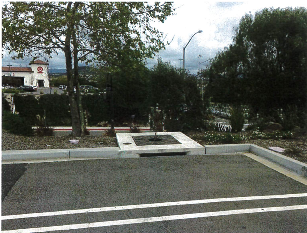
SEWER DRAINS ON SITE, LOOKING SOUTHEAST
