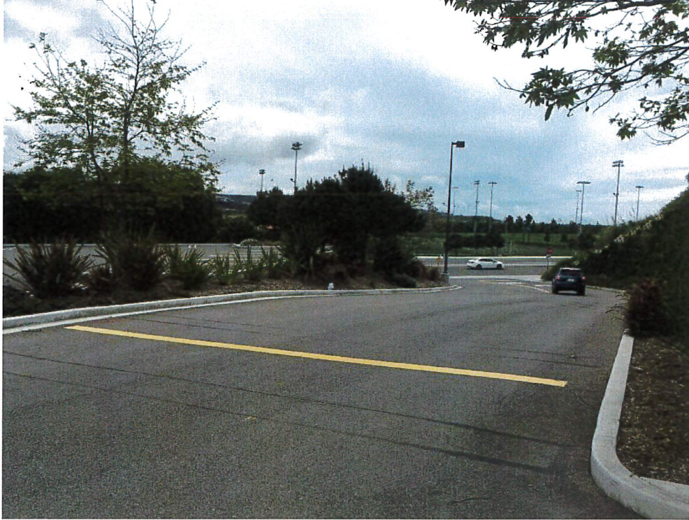
ON SITE ON SECONDARY DRIVEWAY LOOKING TOWARDS AVE. VISTA HERMOSA
