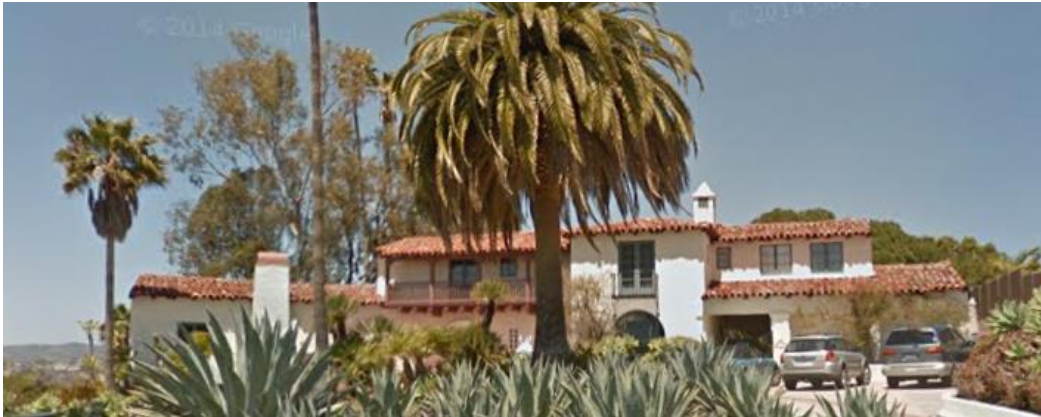
Figure 1 – Existing Site Conditions
