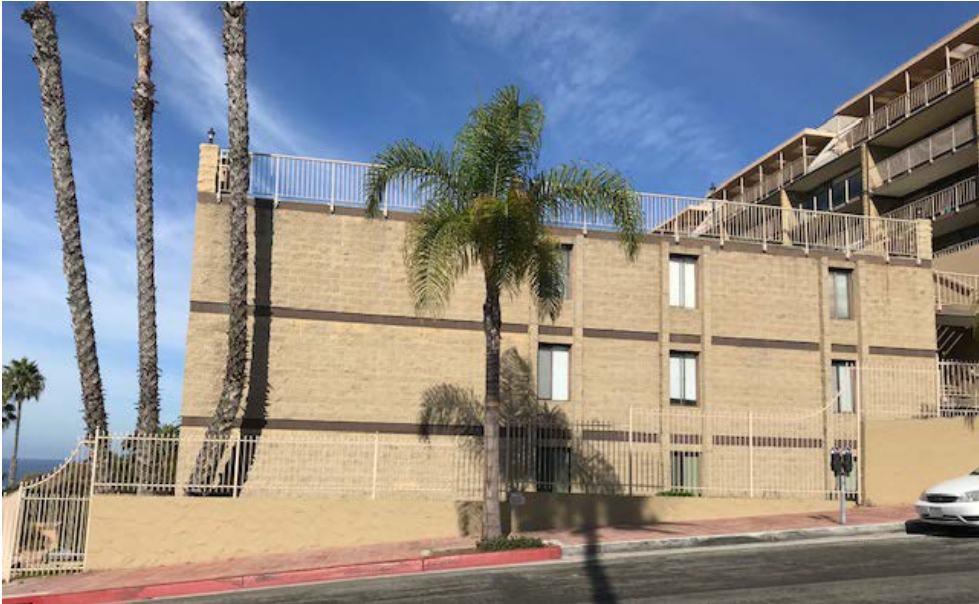
East elevation view from Avenida Del Mar of one of the subject buildings.
