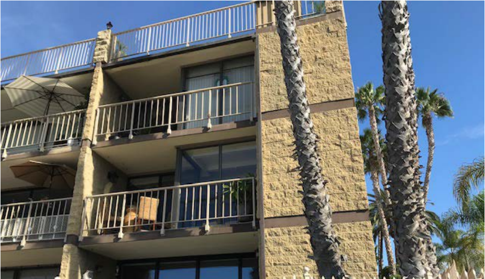
South elevation view from the City's parking lot.
