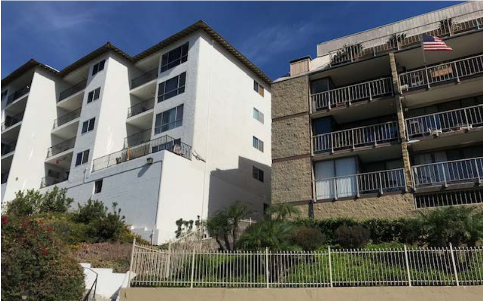
South elevation view from the City's parking lot.
