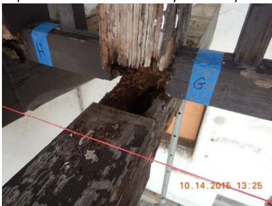
Repair of second floor balcony underway.
