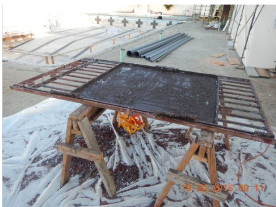
Iron gates refurbished.
