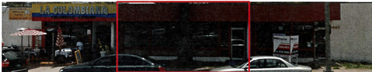
Figure 1a: Existing Building Conditions North Elevations – area of expansion in red
