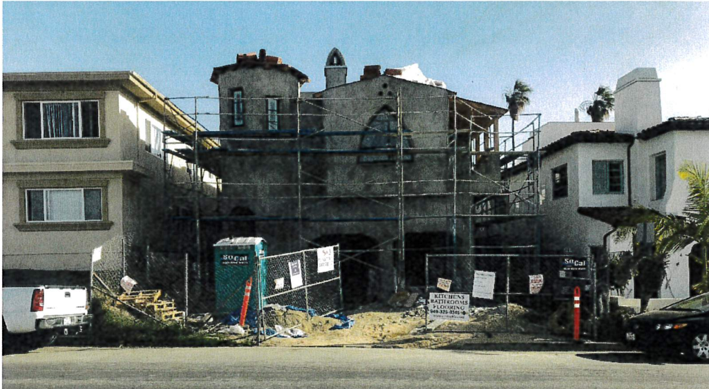
Street view of duplex under construction.
