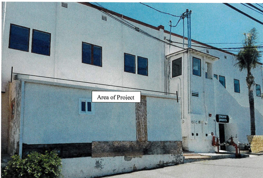
Figure 1: Existing Site Conditions At Rear of Building
