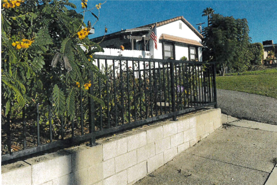
Wrought iron fence above block wall (project site)
