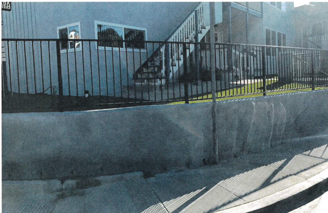
Adjacent wall/fence (southeast of 162 Avenida Rosa)
