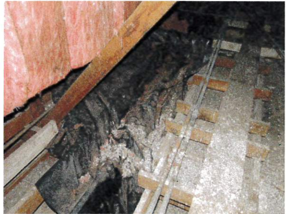
Image 5-14: Tarps used in the theatre attic space in an attempt to reduce water infiltration. 2013.
