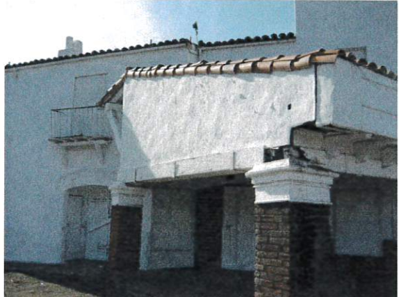
Image 5-5: Decorative brick column with plaster molding at entry portico. 2013.
