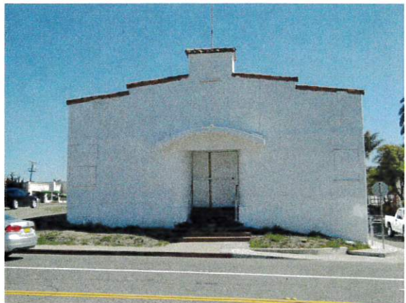
Image 1-5: Main entrance at West facade of Bowling Center. 2013.
