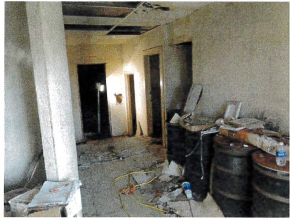
Image 5-19: Bowling Alley office space corridor looking East. 2012.
