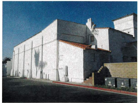
Image 5-8: South façade along Calle Deshecha.. 2013.
