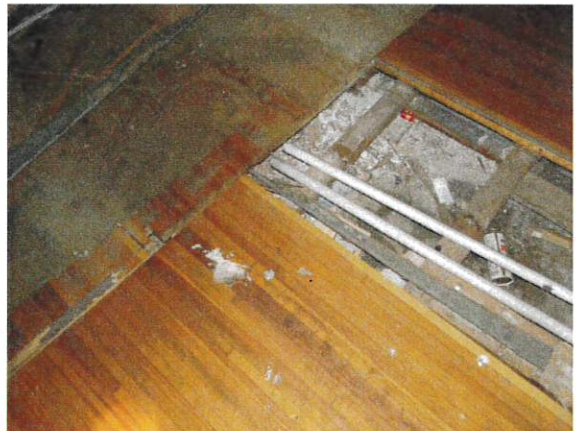
Image 5-18: Remnant of original bowling lane flooring. 2012.
