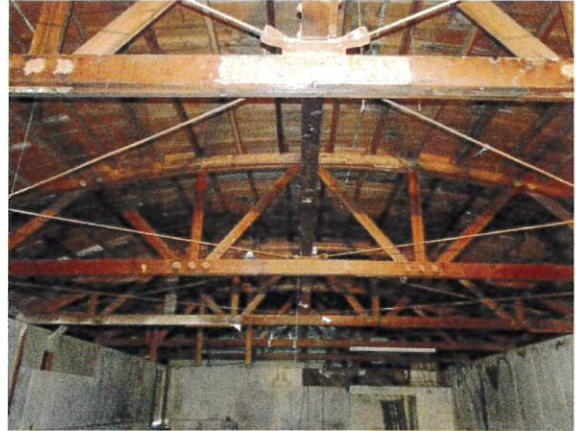
Image 5-17: Main Bowling Alley space looking East. 2012.
