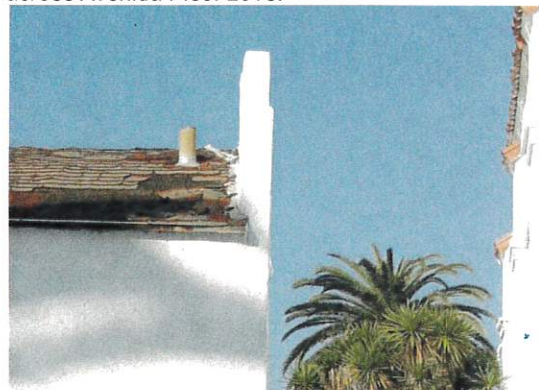
Image 5-15: Typical roofing condition of Bowling Center at East Façade. 2012.
