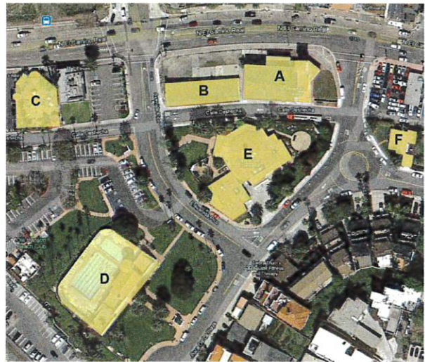
Image 1-2: Site Context – Adjacent Historic Resources:
