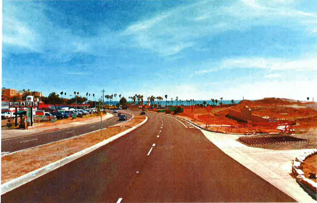
ORIGINAL CORRIDOR VIEW #2
