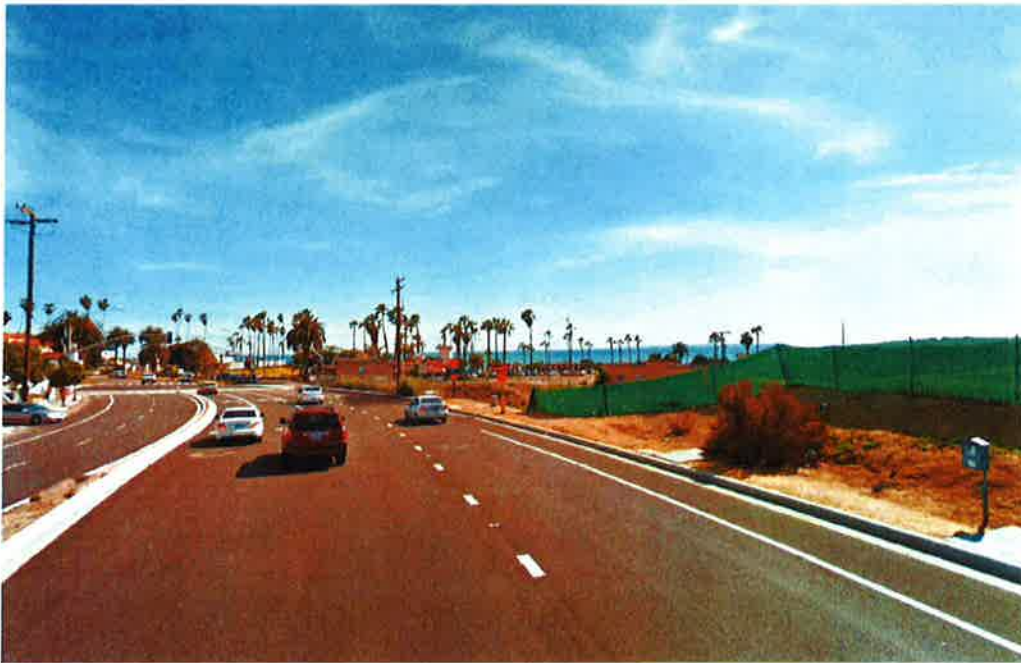
ORIGINAL CORRIDOR VIEW #1
