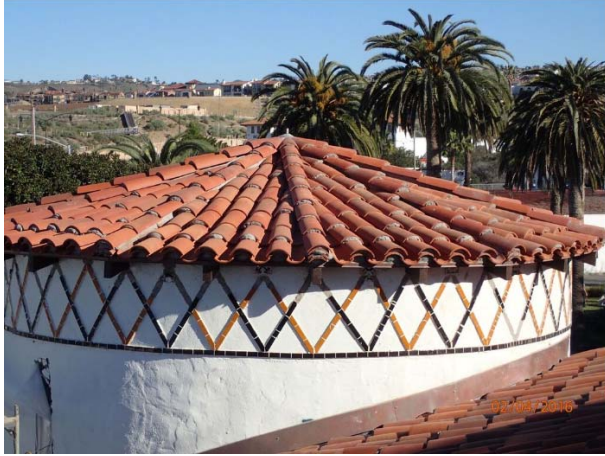
Roof tiles installed.
