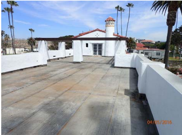
Preparations for deck tile underway.
