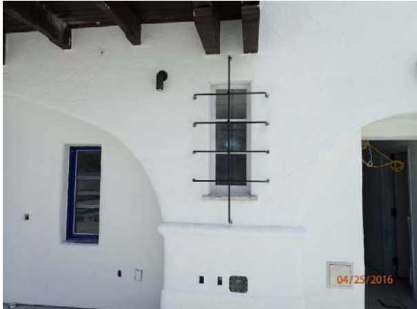
Installation of exterior architectural features underway.
