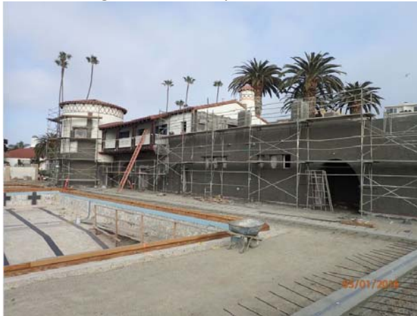
Stucco siding installed and painted.
