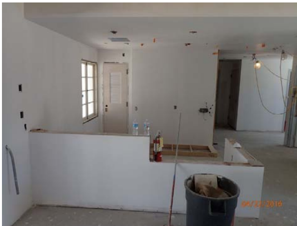
Drywall installed and painted.
