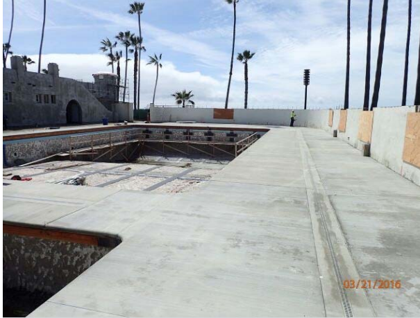
New pool deck poured.
