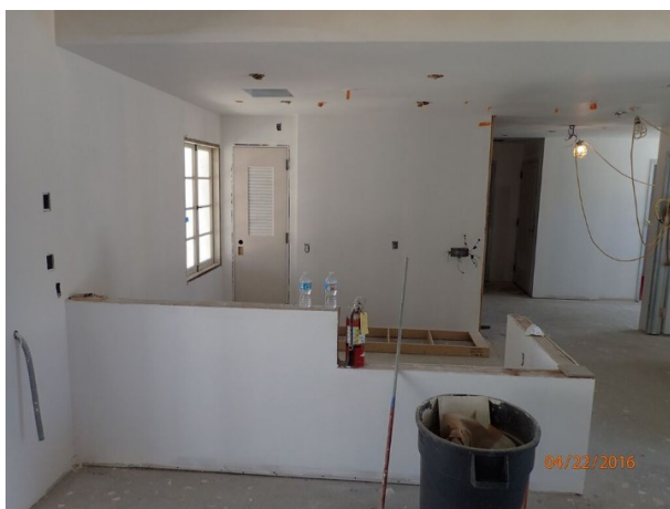
Drywall installed and painted.
