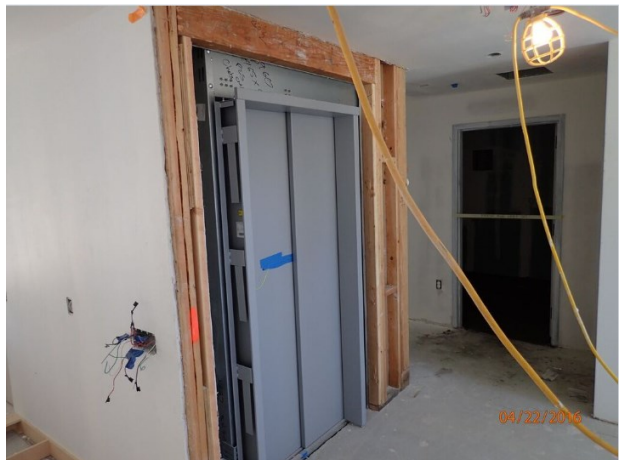
Elevator installation underway.
