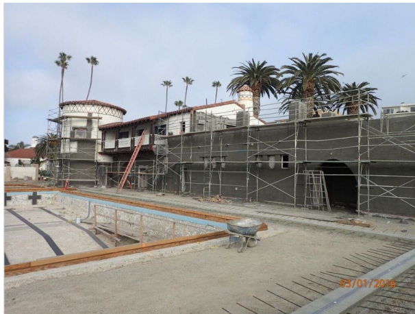
Stucco siding installed and painted.
