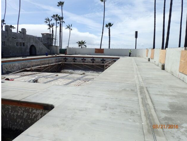
New pool deck poured.
