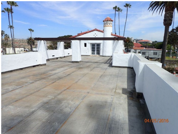
Preparations for deck tile underway.
