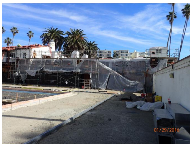
Pool deck trench drains installed.
