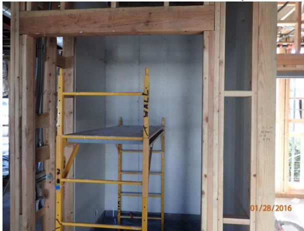
Elevator shaft construction underway.
