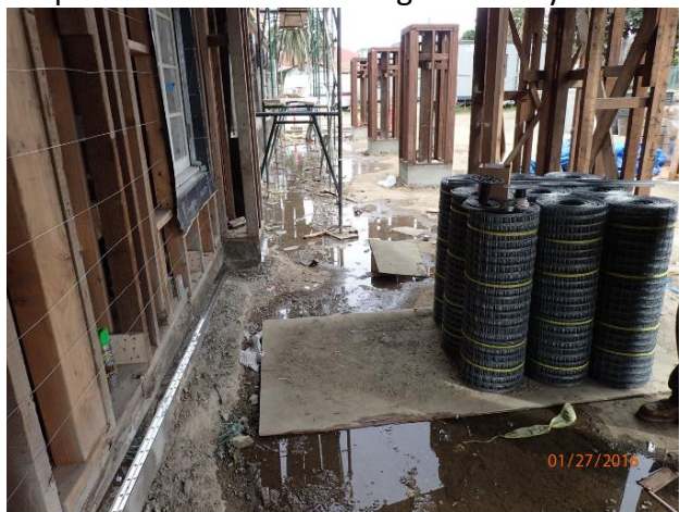
Preparation for stucco siding underway.
