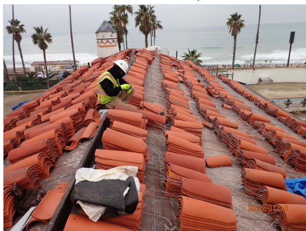
Roof tile installation underway.
