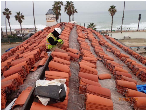
Roof tile installation underway.
