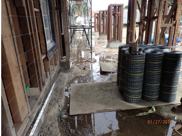
Preparation for stucco siding underway.
