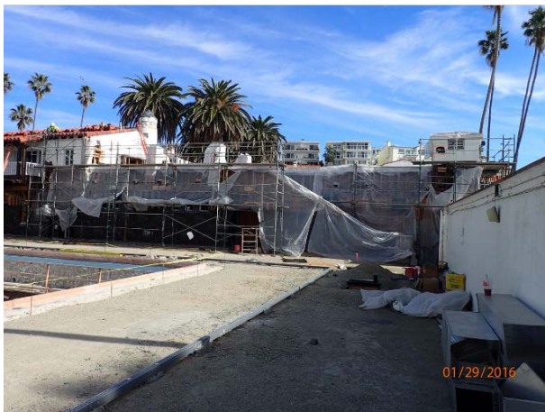
Pool deck trench drains installed.
