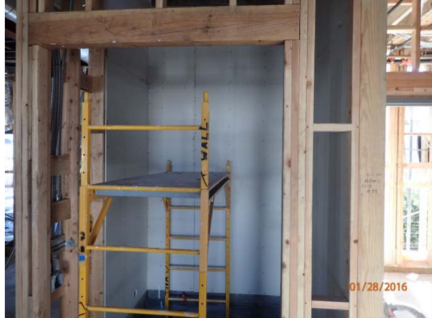
Elevator shaft construction underway.
