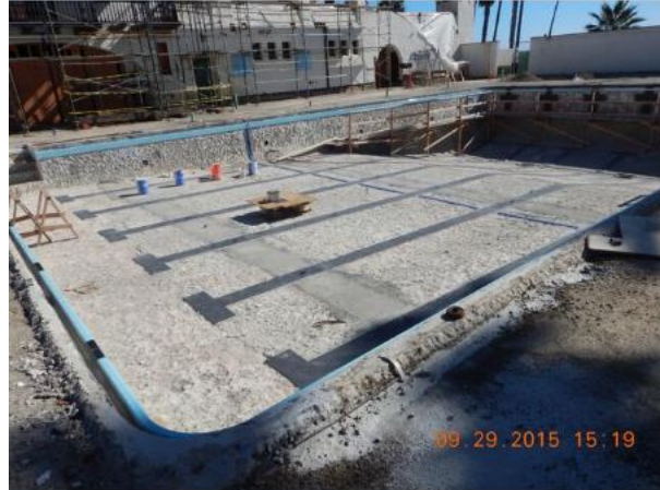
Tile pool markings installed.
