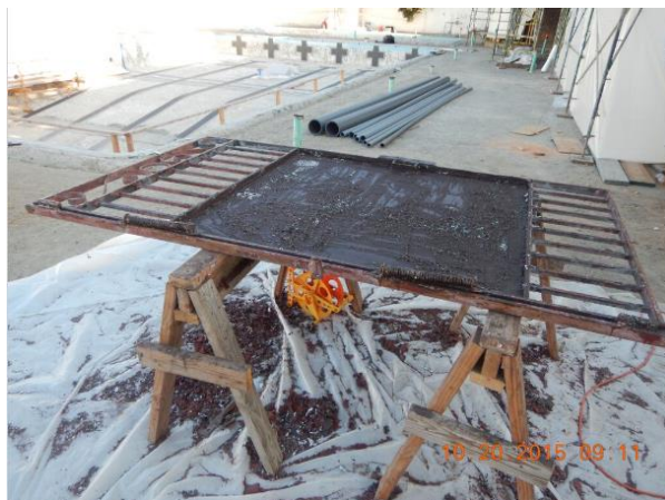
Iron gates refurbished.
