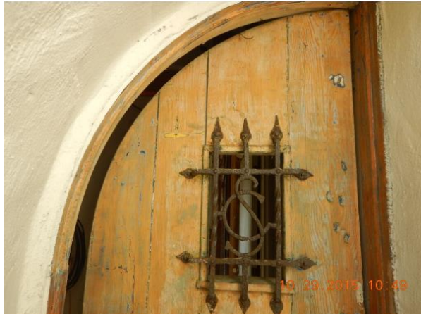
Refurbishment of wood doors and windows underway.
