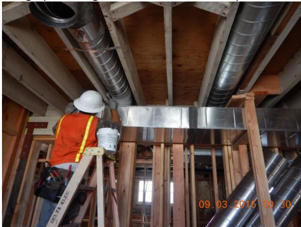
Rough plumbing, electrical, and HVAC systems installed.
