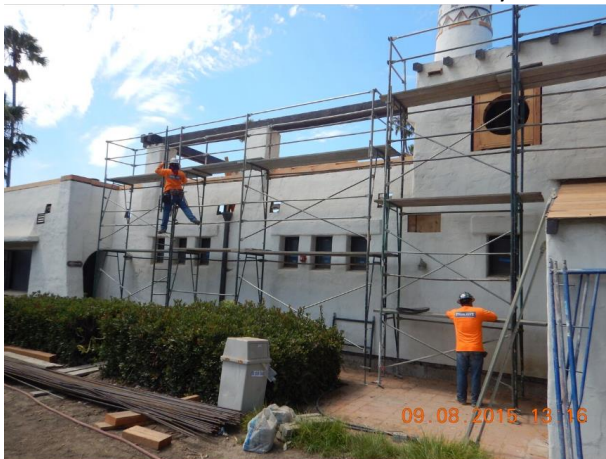
Exterior and historic restoration underway.
