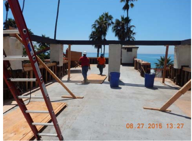
New slab foundation poured.
