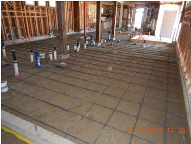
First floor preparations for slab foundation.
