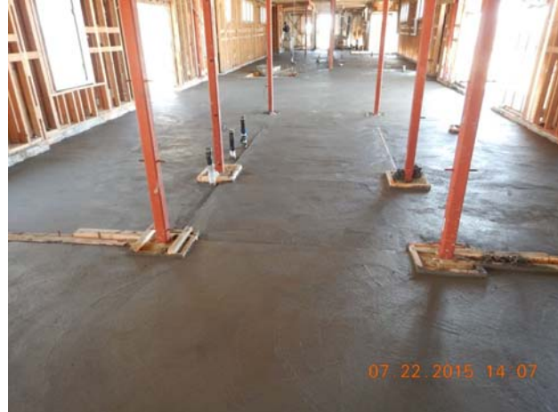
New slab foundation poured.
