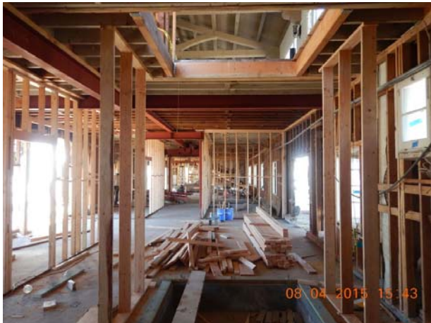
First floor framing underway.
