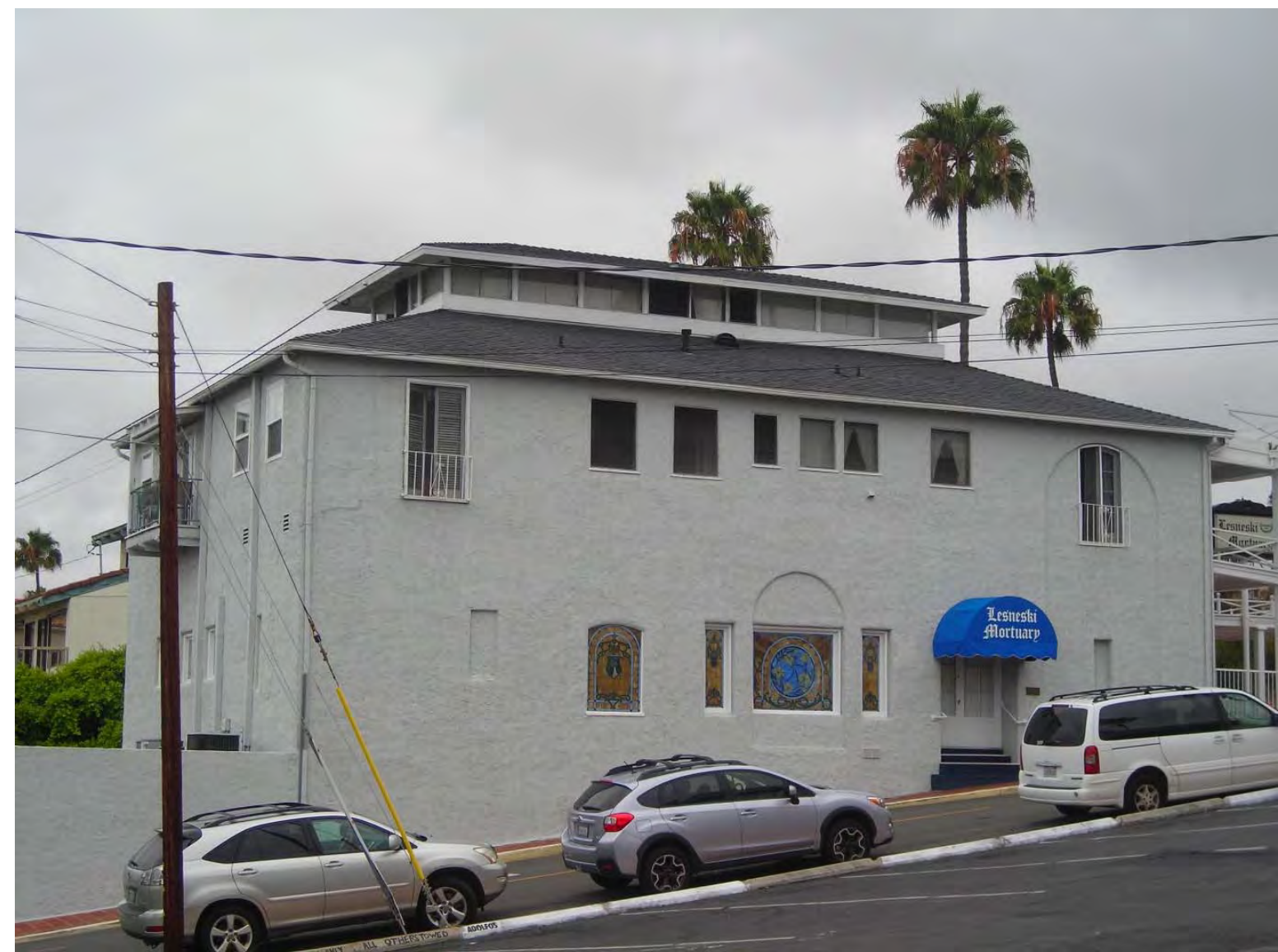
(Facing North from Trafalgar Ln)
