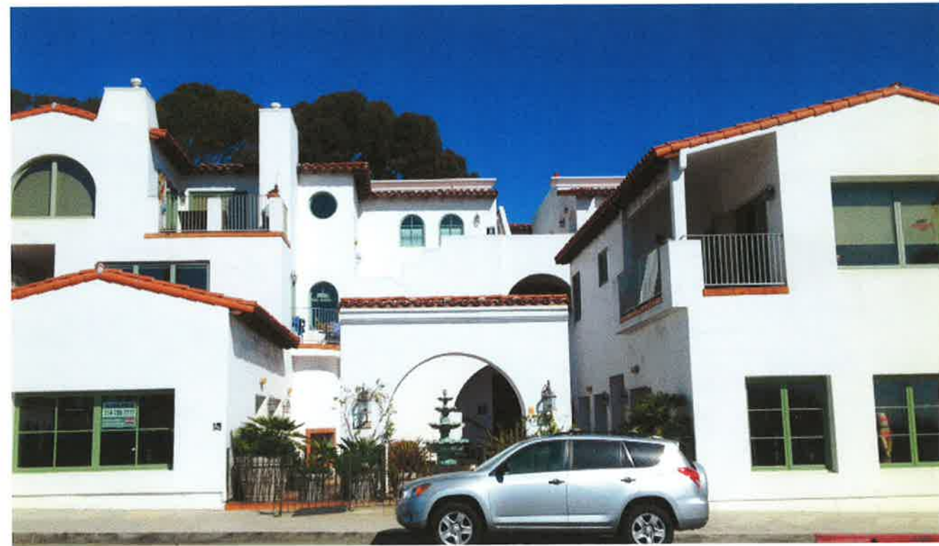
Building Photo: Ave. De La Estrella Facing View
