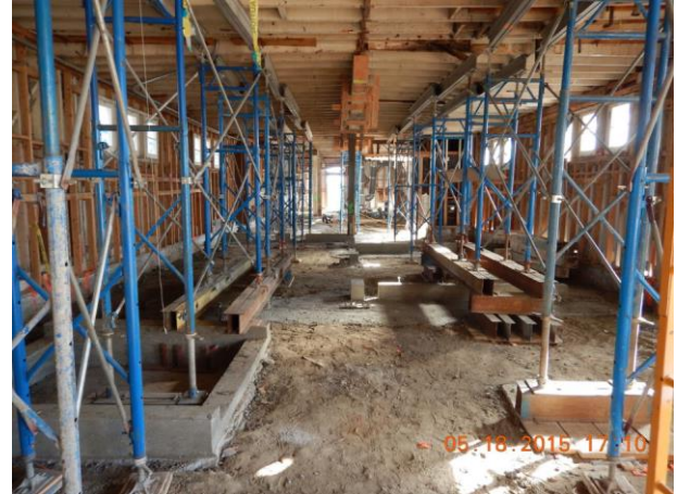
First floor preparations underway and new footings in place for slab foundation.
