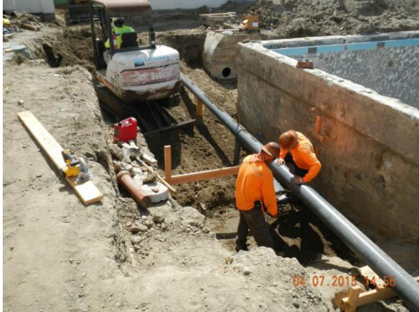
Pool systems improvements underway.
