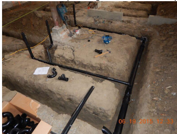
First floor interior plumbing installation underway.
