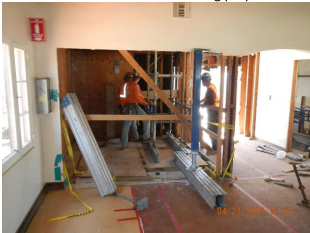
Second floor elevator location being prepared.
