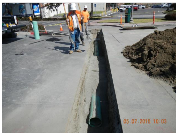
Installation of site drainage and sewer improvements underway.
