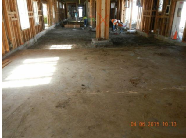
First floor preparations underway and new footings in place for slab foundation.
