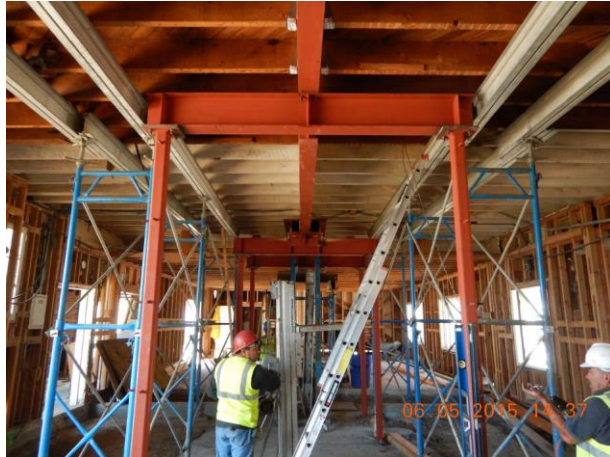
Replacement structural support beams and posts installed.
