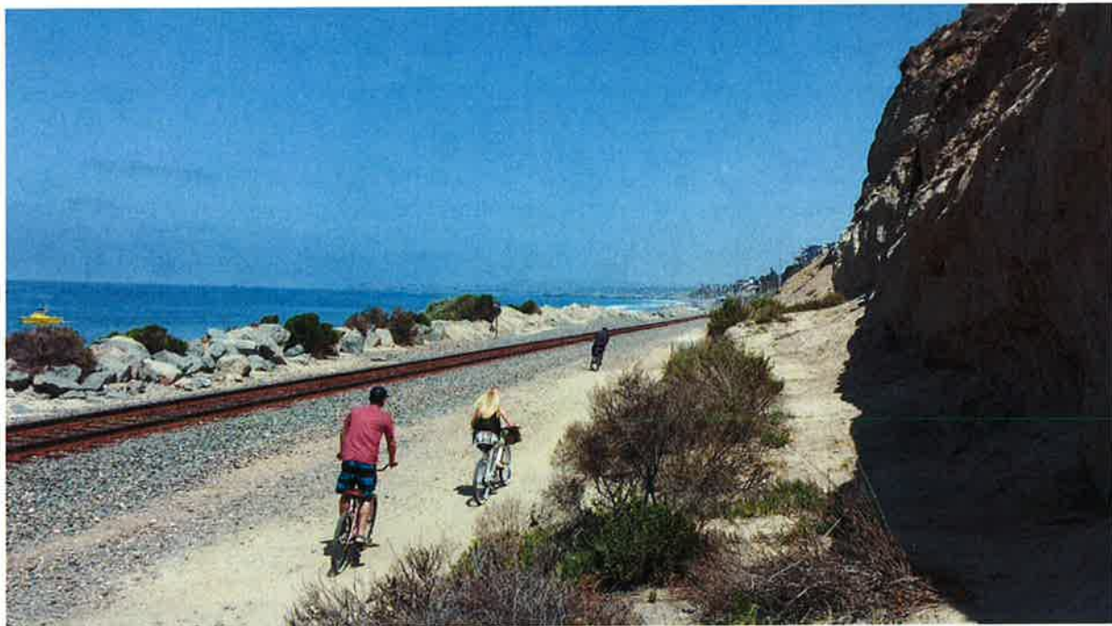
Photo 4: This photo demonstrates how the space between the bluff and railway narrows significantly, thereby placing people within an arm's reach of passing trains. Adding to the risks are the jagged, golfball-sized rocks stabilizing the railbed, which creates a shifty surface for pedestrians and bicyclists. Especially after rainfall, puddles several inches deep form on the inland side of the tracks, so people walking and biking often travel over the rocky rail bed, which presents additional risks of tripping/falling in close proximity to trains.
