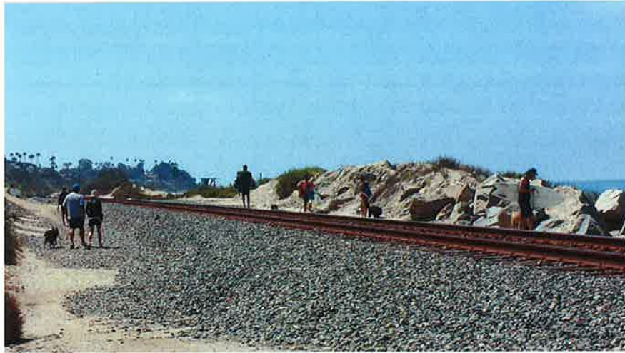
Image 1: Pedestrians within the Railroad ROW South of Avenida Calafia
