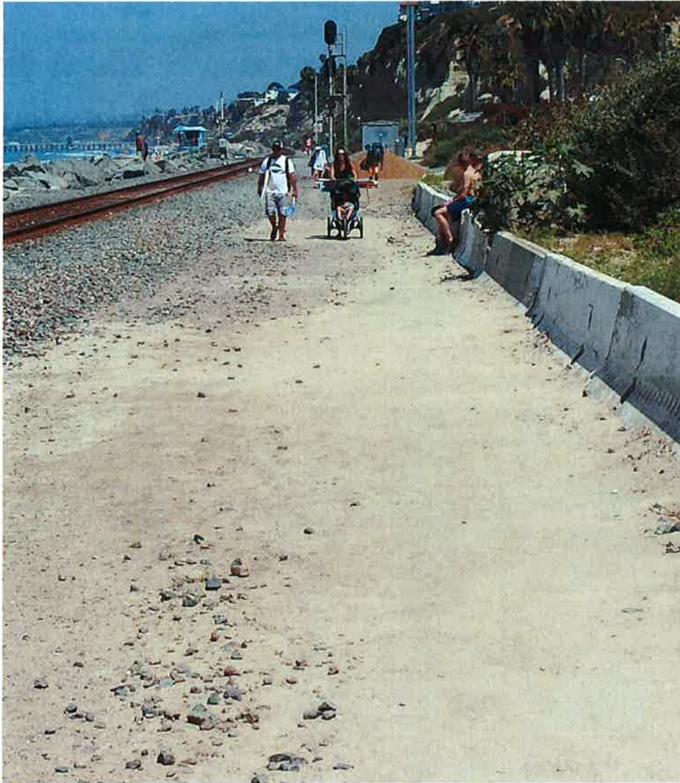
Photo 5: This photo demonstrates the jagged, golfball-sized rocks stabilizing the railbed, which creates a shifty surface for pedestrians and bicyclists. To protect trains from crumbling sandstone and rocks, railroad maintenance crews added temporary concrete k-rail barriers between the sandstone cliffs and the rail bed. The barriers narrowed the navigable path, safeguarding trains but increasing risks to trespassers who have been using the rail bed for decades.
