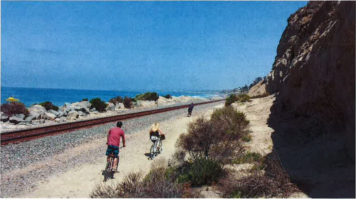
Photo 4: This photo demonstrates how the space between the bluff and railway narrows significantly, thereby placing people within an arm's reach of passing trains. Adding to the risks are the jagged, golfball-sized rocks stabilizing the railbed, which creates a shifty surface for pedestrians and bicyclists. Especially after rainfall, puddles several inches deep form on the inland side of the tracks, so people walking and biking often travel over the rocky rail bed, which presents additional risks of tripping/falling in close proximity to trains.
