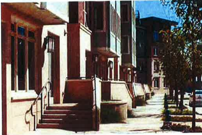
To help ensure privacy and safety for residents, some doorways were elevated and store windows were reduced to a more residential scale. (JHP)
