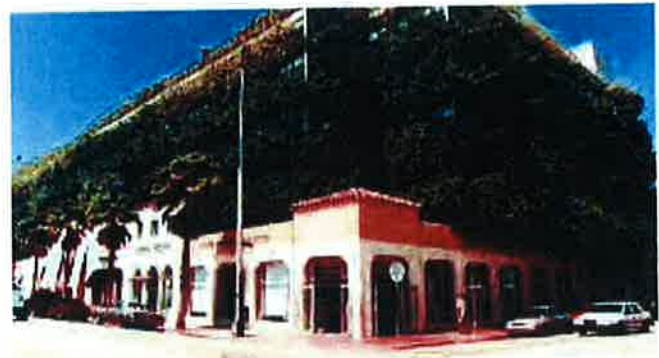
The parking garage at Seventh and Collins, Miami Beach, Florida.
