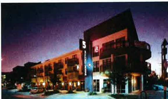
The problem of small initial retail demand was solved by reducing the depth of retail space to 30 feet (9 m), less than half the building depth, with residential units filling the other half and opening onto the internal courtyards. The shallow depths also shielded the parking structure from view. (Mark Olsen)
