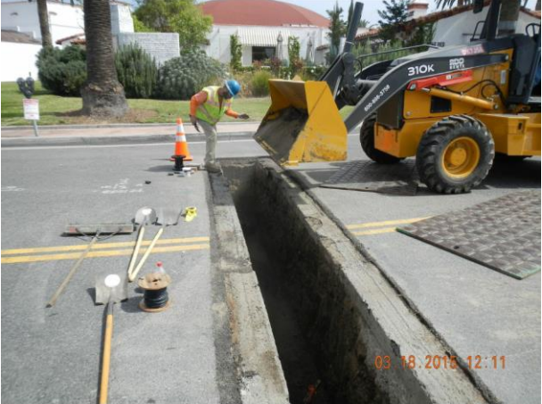
New Water Line Installed
