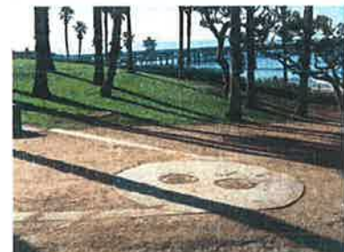
Underground unit installed at Parque Del Mar (next to Pier Bowl parking lot).
