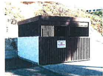
Covered trash enclosure at Calafia.
