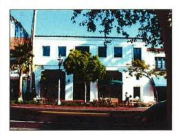
Henry Lenny Design Guidelines; Wall Openings. Windows and doors should be set toward the interior allowing the wall thickness to be revealed on the exterior of the building. Walls should be no thinner than 12". An 18" wall is ideal.
