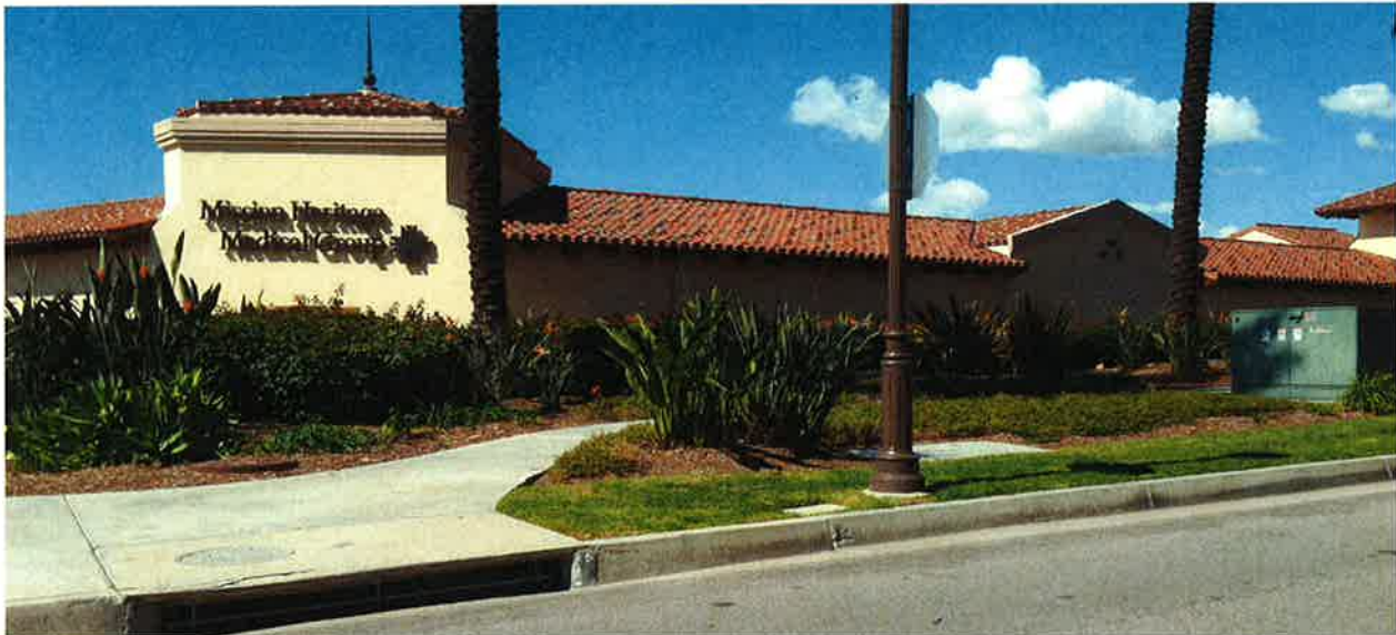
Shops 3, East Elevation facing Avenida Talega
