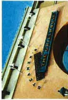
Pin set flat cut out letters and aluminum panel with flat cut out letters with gooseneck lamp illumination
