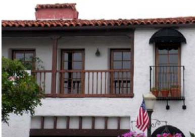
Spanish Colonial Revival details characterize this commercial building at 122-124 Avenida Del Mar.
