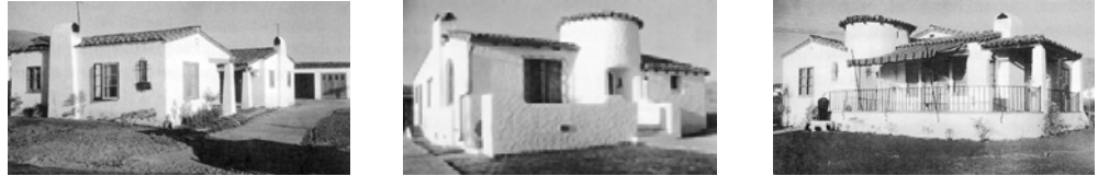
Ole Hanson-era residences exhibit typical Spanish Colonial Revival elements, including white stucco walls, hand-made clay roof tiles, wood-frame windows, and wrought-iron ornamentation. (Walker, 77).
