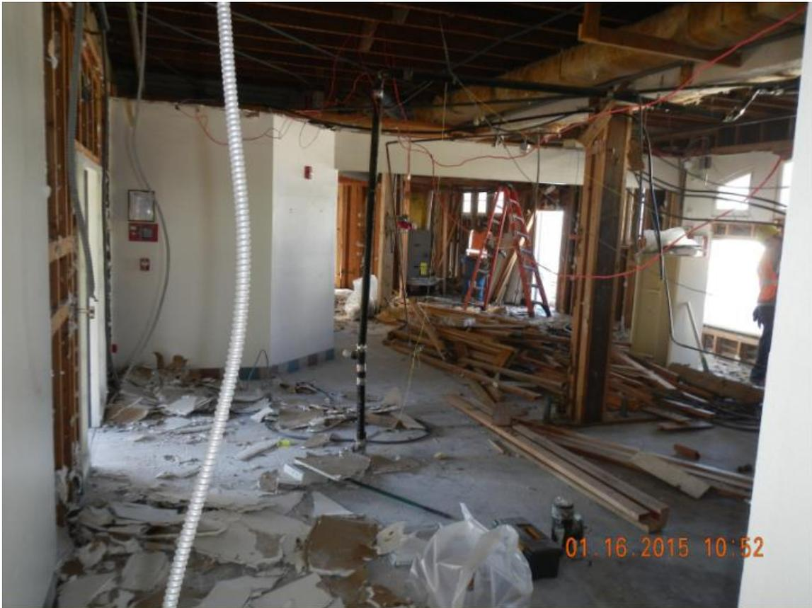
Over the course of 80 years many types of construction methods were discovered that are very different to today's current standards. For example, notice the original white supporting column that had been cut and is off-set on the photo on the left, and the removal of supporting members and unusual bracing that was used.
