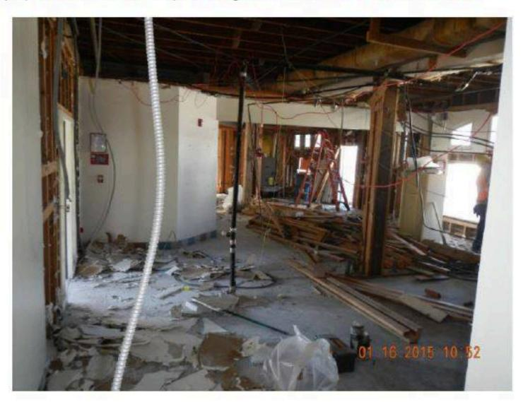
Over the course of 80 years many types of construction methods were discovered that are very different to today's current standards. For example, notice the original white supporting column that had been cut and is off-set on the photo on the left, and the removal of supporting members and unusual bracing that was used.
