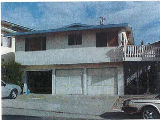
Before: downtown multi-family apartments at 255 Avenida Victoria
