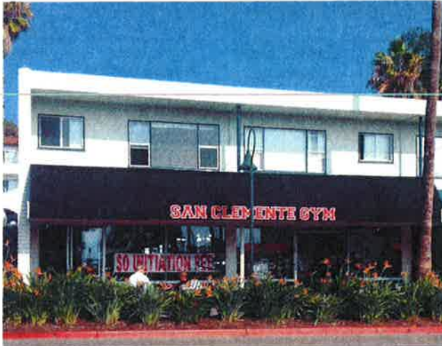
After Photo: Awning compliments the building and adds more visible signage to a busy Downtown thoroughfare, freshens and updates the business.
