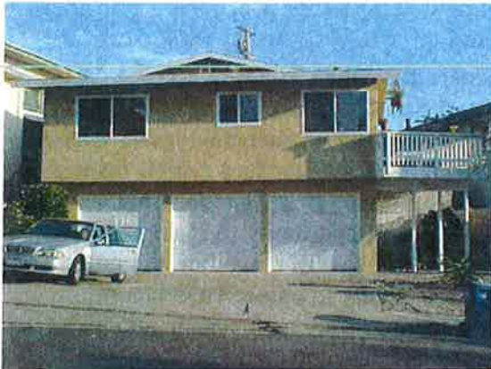
After: newly renovated and painted apartment
