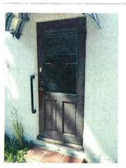
Replace the deteriorated door with a traditionally designed Spanish door.
