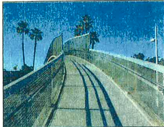
Pedestrian bridge over I-5
