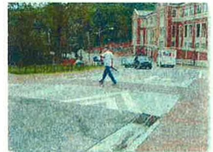
Raised crosswalk: University of North Carolina, Chapel Hill, NC (Credit: Ryan Snyder)
