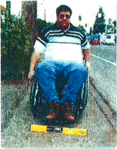
Steep cross slopes create difficulties for wheelchair users (Credit: Michael Ronkin)
