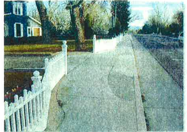
Routing sidewalks around driveway ramps maintains a flush surface (Credit: Dan Burden)
