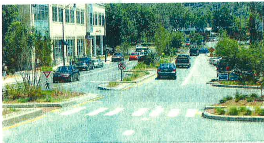
Curb extensions and medians make crossing multi-lane streets safer and more manageable (Credit: Dan Burden)
