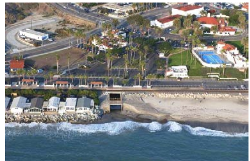
Aerial view of North Beach 1 .
