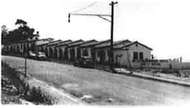
The 1947 Beachcomber Motel is recommended for designation as a local landmark.
