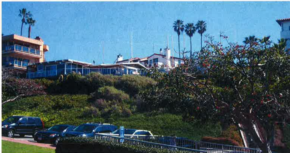
Image 3: View of the project site from Linda Lane Park. The highest point of the proposed structure is consistent with the two neighboring properties.
