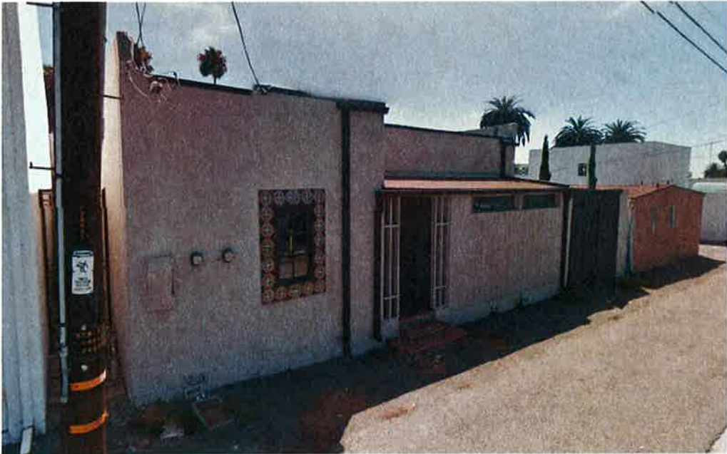
Image 2: Rear façade as seen from Los Obreros Lane and Calle de Los Molinos
