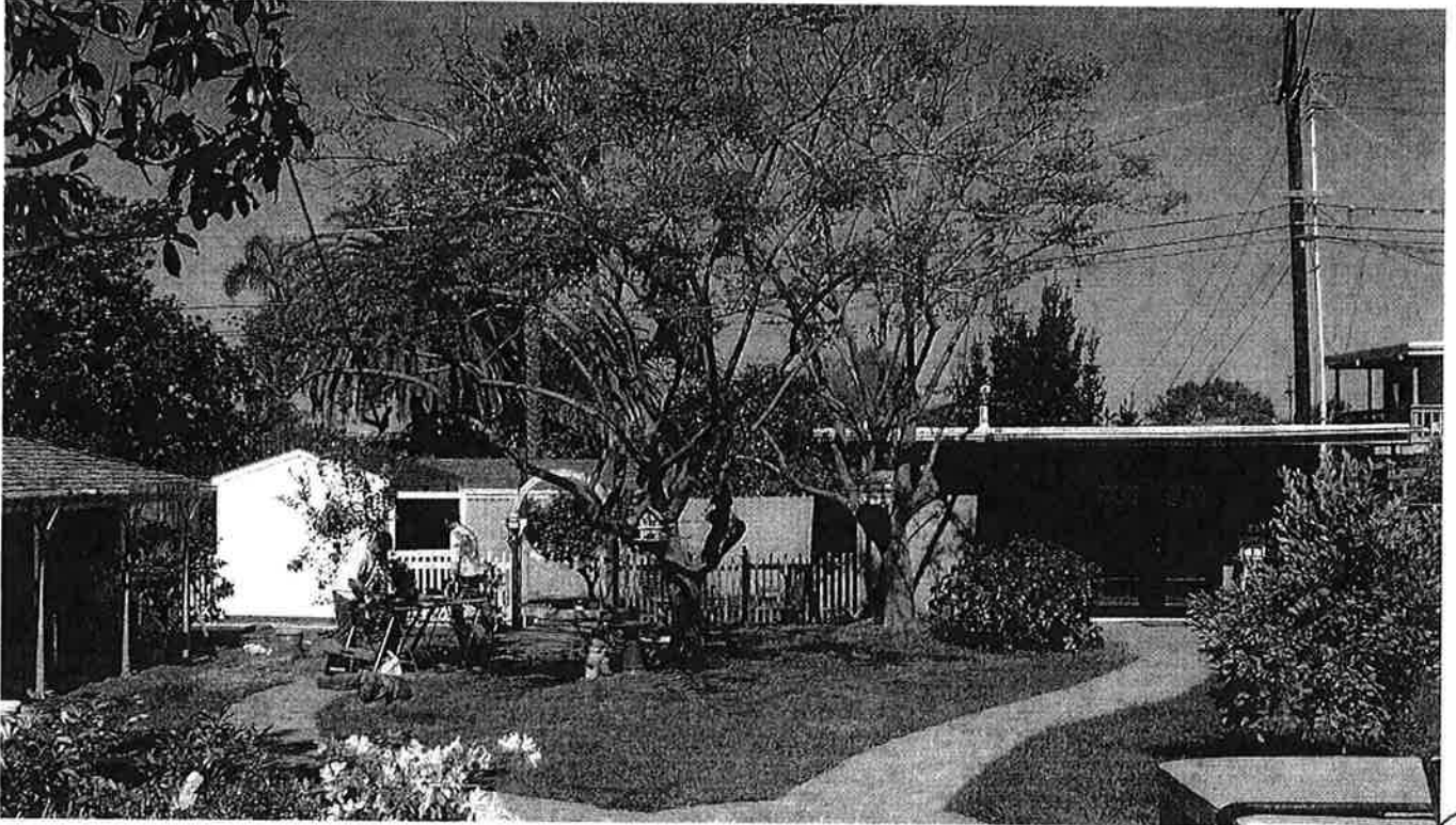
ROOF OF HISTORICAL STRUCTURE
