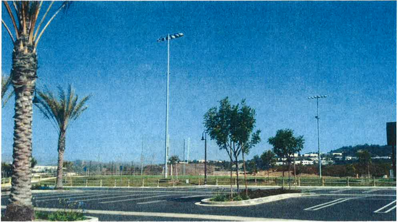
Cellular Light Pole Site (View 3).
