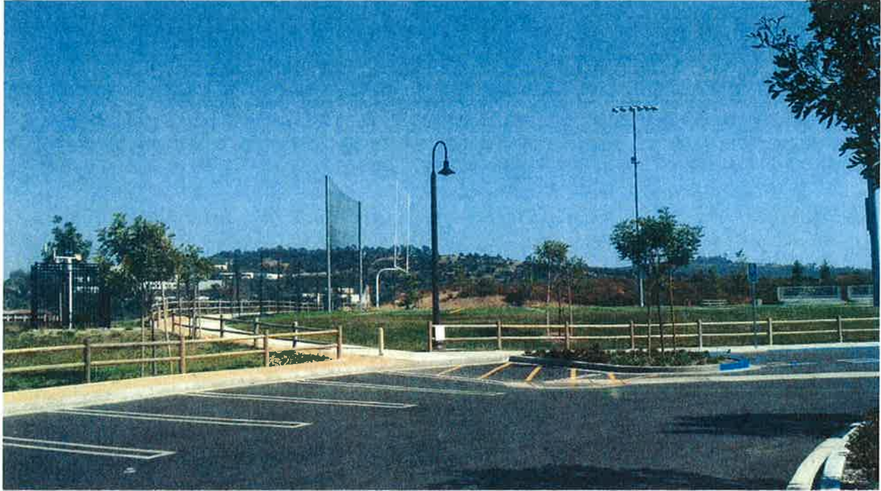
Cellular Light Pole Site (View 1).
