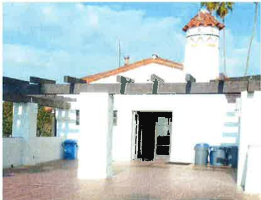
EXISTING VIEW OF WEST ELEVATION AT WEST DECK
