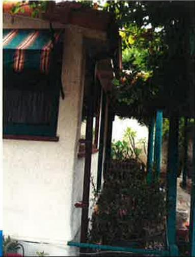
Replace the non-traditional gutters with copper gutters.
