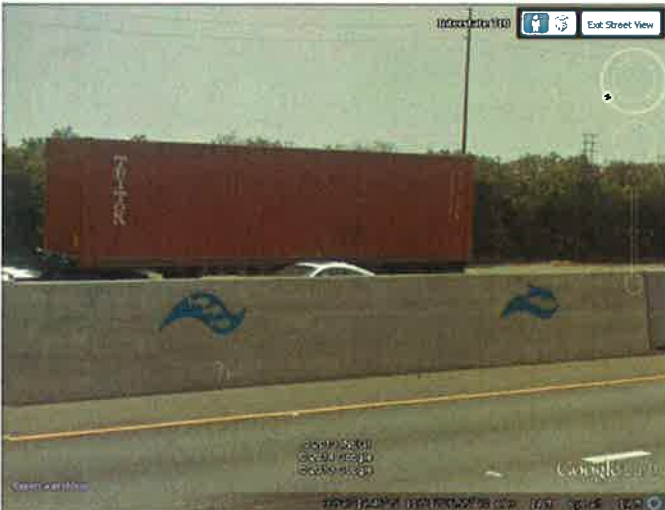
Sand blasted and painted barrier on I-710
