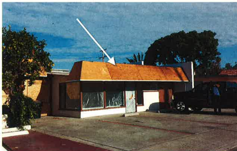
Figure 1 – Roof element removal at 144 Avenida Serra
