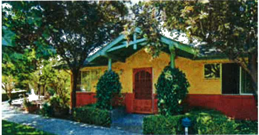
Hendley Circle Apartments – Supportive SRO Housing in Burbank Photo courtesy of Burbank Housing
