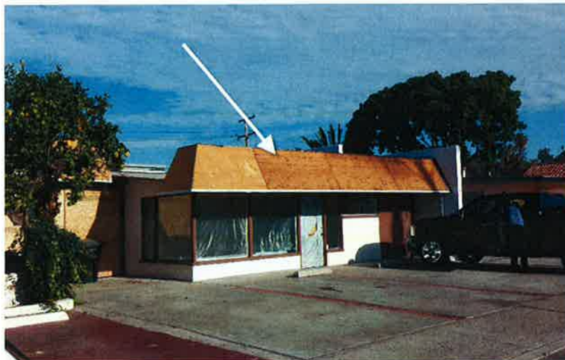
Figure 1 – Roof element removal at 144 Avenida Serra
