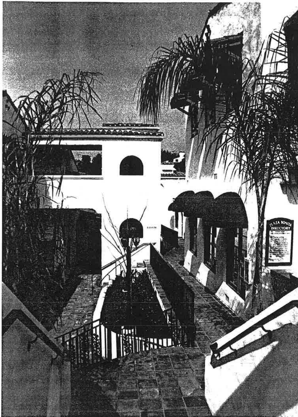
Plaza Bonita. El Camino Real. Successful example of a courtyard used as focus for a commercial center.
