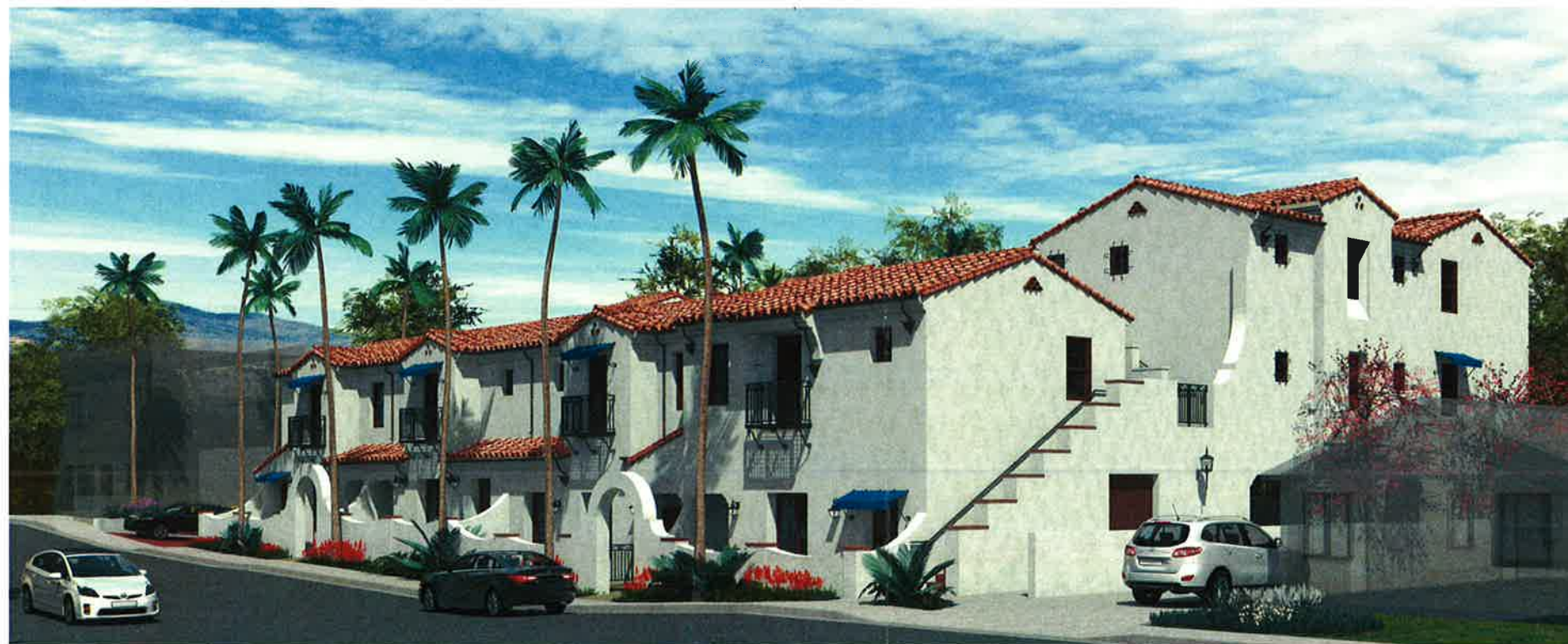
SOUTH-WEST STREET VIEW
