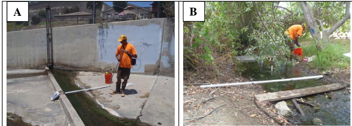
Figure 5-4. Stream Rating and Flow Monitoring at Site A (upstream) (A) and Site D (downstream) (B) in the Bioswale Effectiveness Assessment
