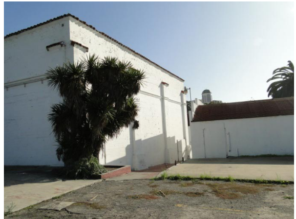
Image 5-9: West theatre façade showing theatre egress path. 2013.
