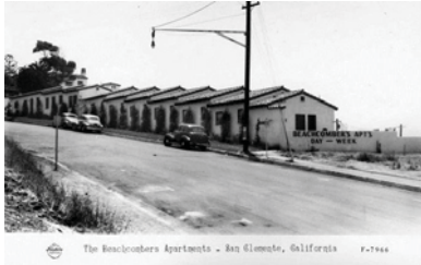
The 1947 Beachcomber Motel is recommended for designation as a local landmark.
