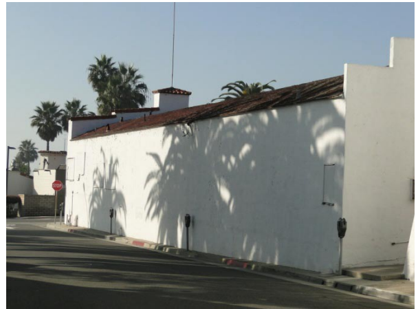
Image 1-6: South façade of Bowling Center. 2013.
