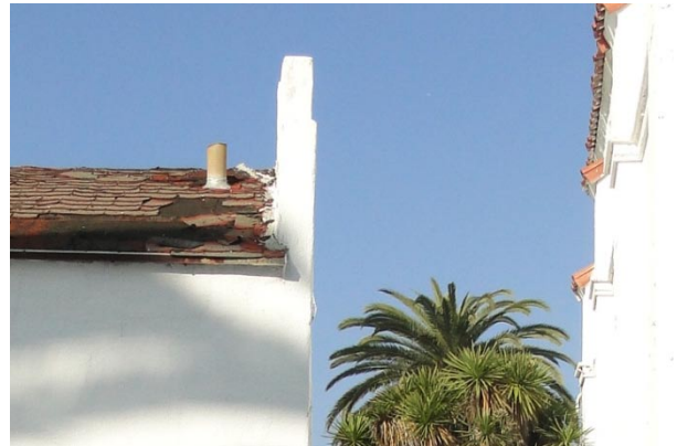
Image 5-15: Typical roofing condition of Bowling Center at East Façade. 2012.
