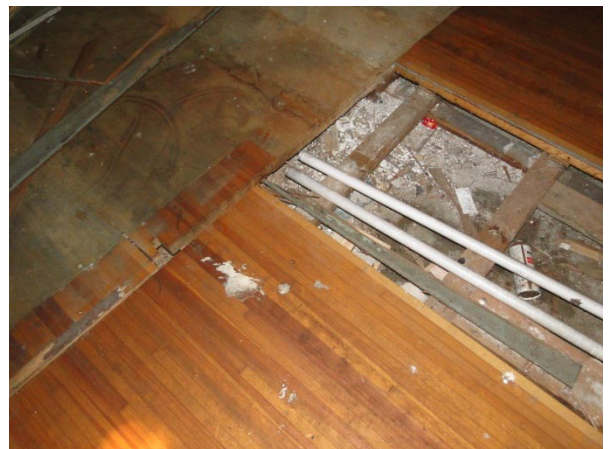
Image 5-18: Remnant of original bowling lane flooring. 2012.
