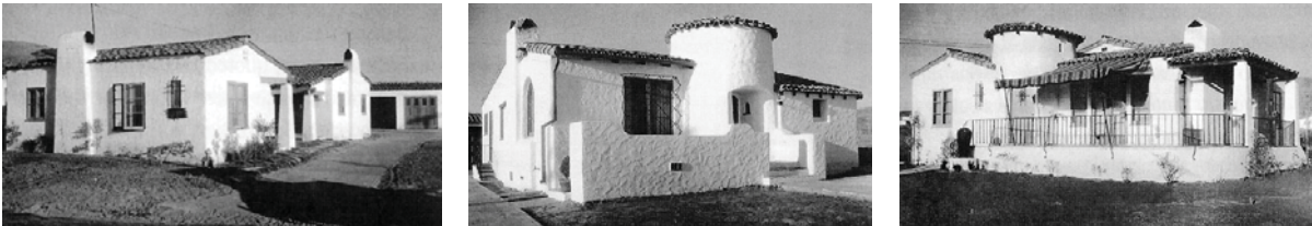
Ole Hanson-era residences exhibit typical Spanish Colonial Revival elements, including white stucco walls, hand-made clay roof tiles, wood-frame windows, and wrought-iron ornamentation. (Walker, 77).
