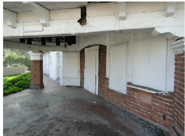
Image 5-6: Various brick elements at entry portico. 2013.
