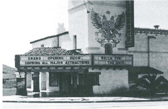
Image 3-1: View of Miramar Theatre, 1938. Source: San Clemente Historical Society.
