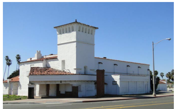
Image 5-2: Partial North and East façade along North El Camino Real. 2013.
