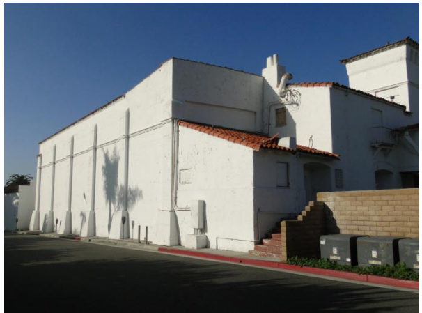
Image 5-8: South façade along Calle Deshecha.. 2013.
